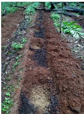
Filling up of trench with compost and manures
