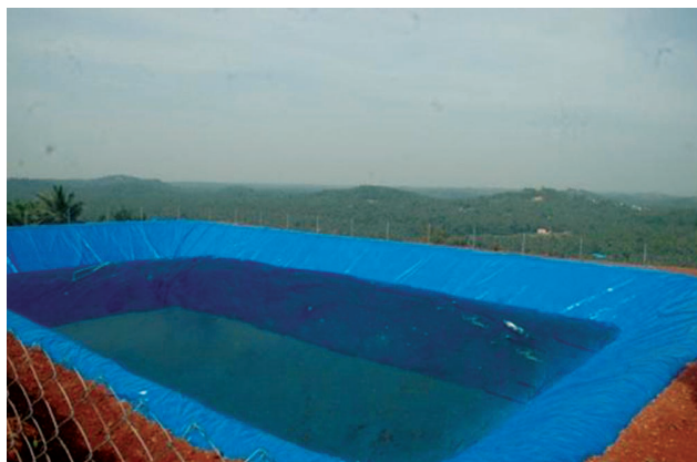
Water harvesting structure
