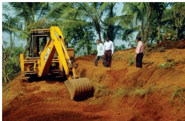
Terracing of land in progress
